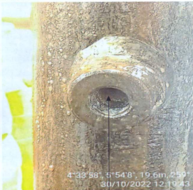
SPILL POINT (REMOVED PLUG)
