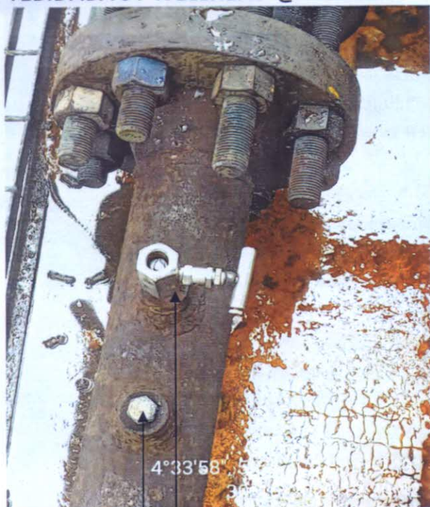
PLUG EXAMPLE ON THE WELLHEAD BEFORE REMOVAL
